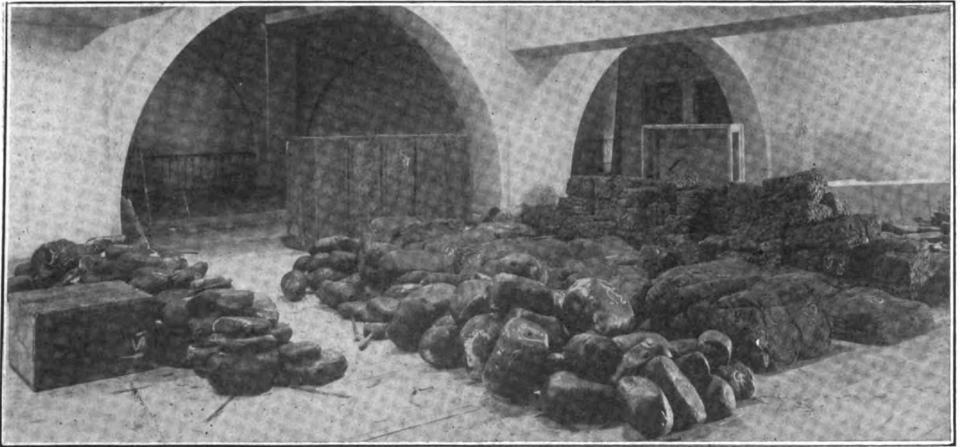
In the foreground are heaps of up-river fine, which is coarse, and in the background heaps of up-river coarse, which is fine
